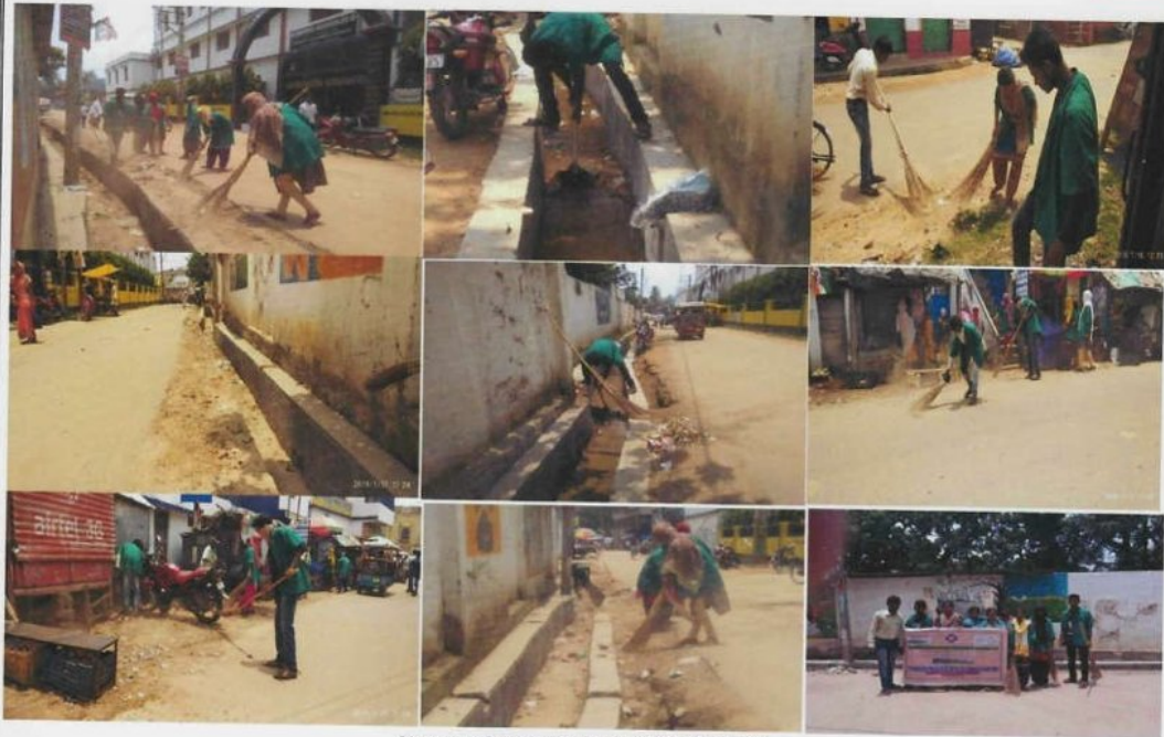
Pictures of Road & Drainages Cleaning 2.0
